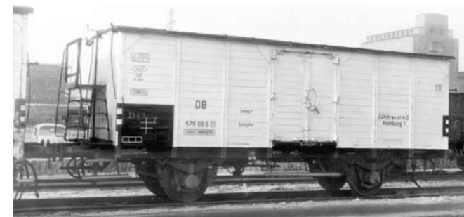
Prototype of the Z-gauge Annual Car 2013: DB's G 10 with heat insulation installed was working for the company Kühltransit AG in era III.
